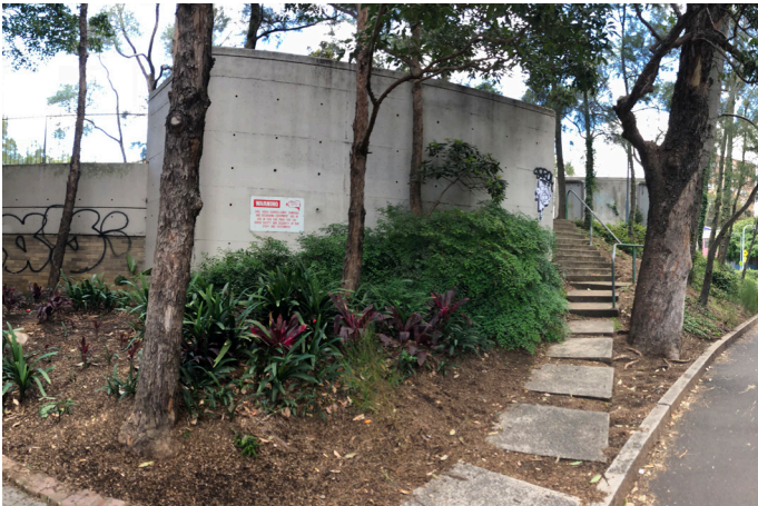
Existing stair entry to Lawrence Hargrave Reserve
